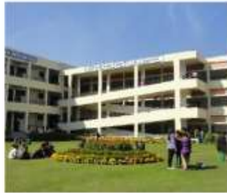
Well ventilated building structure
